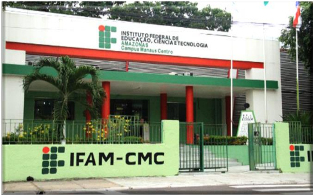
Figura 2-Fachada Principal do IFAM Campus Manaus – CMC
